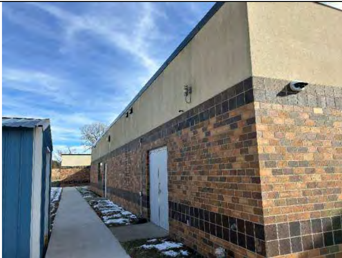
Elevation 5: Repair thin EIFS seal wall penetrations.
