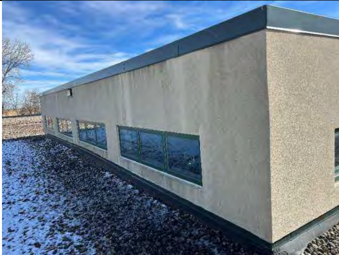
Elevation 13: EIFS is thin and needs cleaning.
