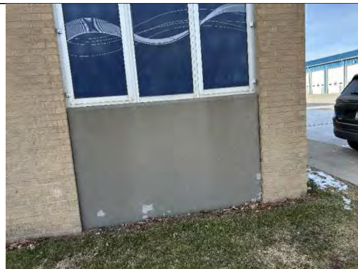
Elevation 3: EIFS below windows failing.
