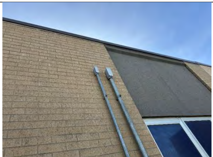
Elevation 3: Sealant needed at conduit penetrations.
