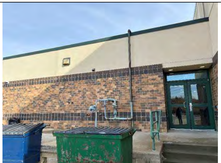
Elevation 6: Repair EIFS, paint gas pipe and railing.
