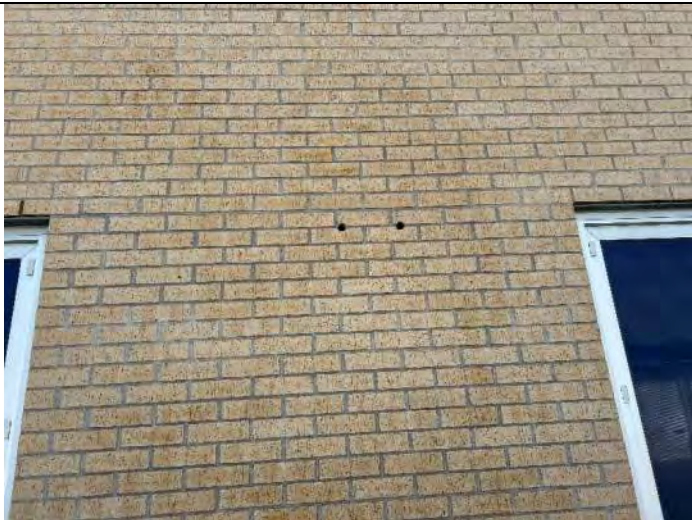
Elevation 4: Grout holes in brick.
