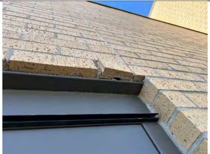
Elevation 11: Repair broken brick above door.
