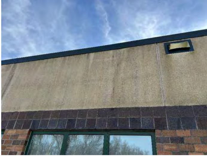
Elevation 3: Repair thin EIFS, reseal control joints.
