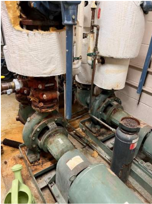
Figure 1 – Geothermal Loop Pumps
