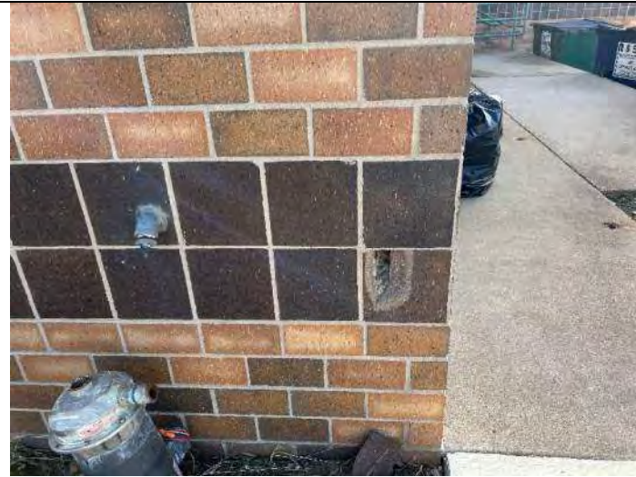
Elevation 5: Repair brick with broken face.
