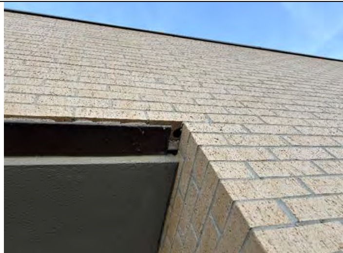
Elevation 4: Repair mortar at entry opening.
