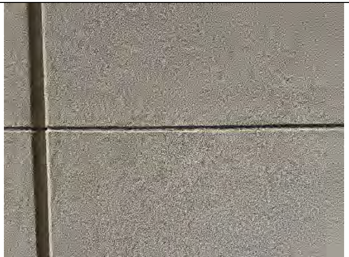
Elevation 12: Control joints need resealed.
