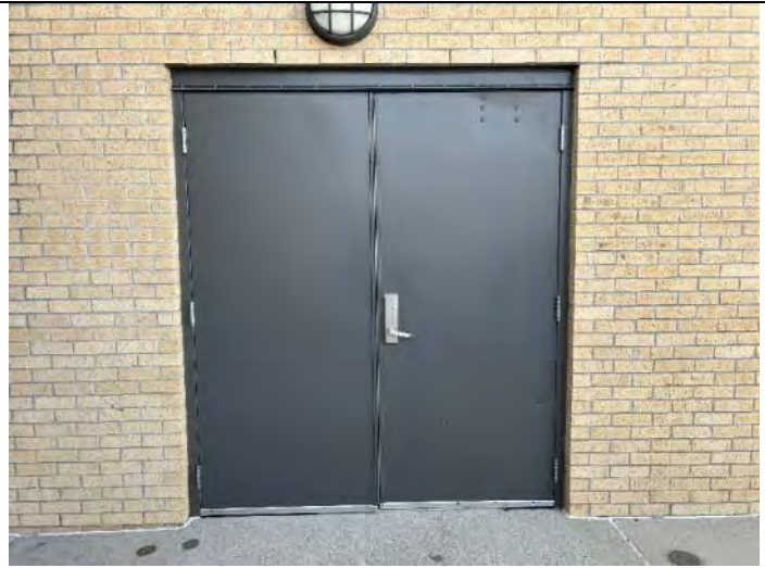
Elevation 4: HM door into weight room needs replaced.
