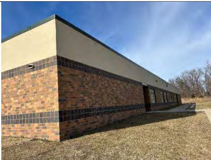
Elevation 2: Need EIFS repair and cleaning
