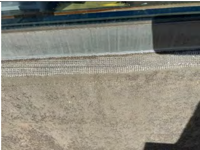
Elevation 9: EIFS needs repair.
