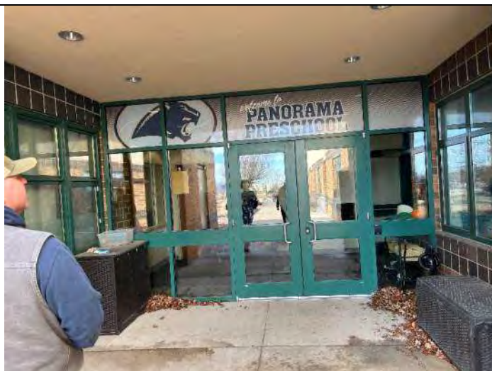
Elevation 9: Reseal windows all around.
