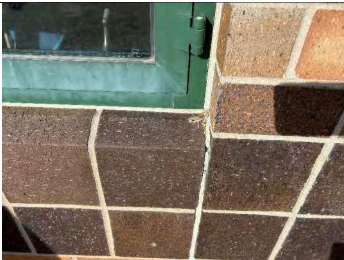
Elevation 1: Control joint needs mortar removed and sealant installed.
