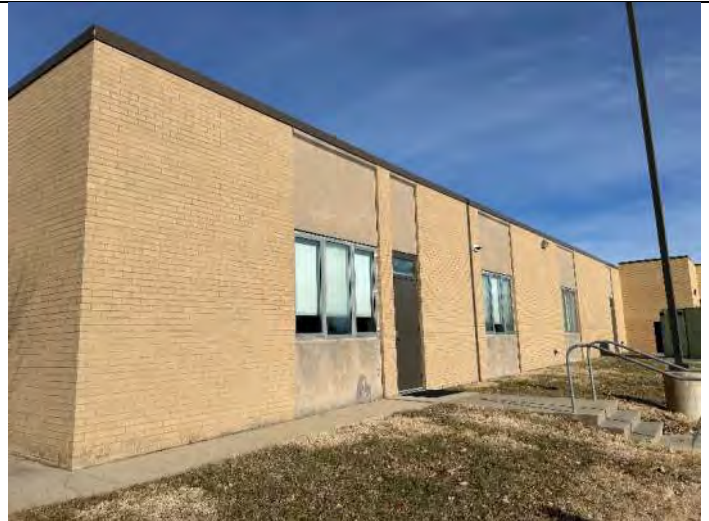
Elevation 9: EIFS needs repair, reseal windows & doors.
