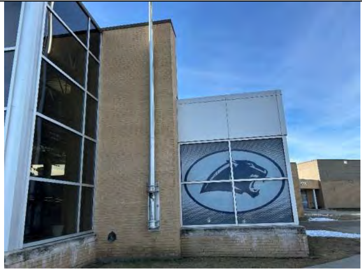
Elevation 12: Clean and seal brick and sill.
