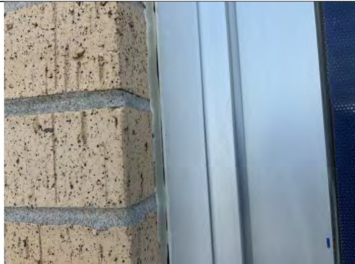
Elevation 4: Window sealant failed typically.
