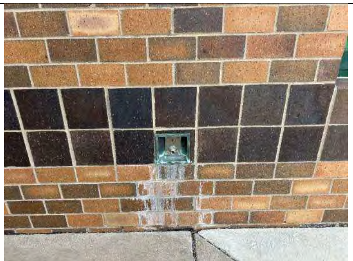
Elevation 9: Clean lime off brick.
