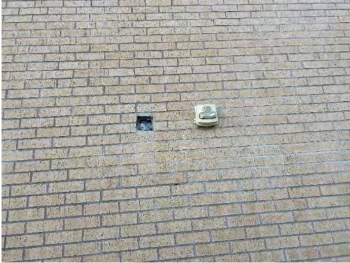
Elevation 12: Electrical box needs a cover.
