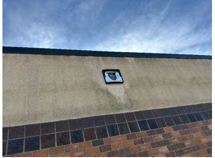
Elevation 3: Replace missing lense and bulb.
