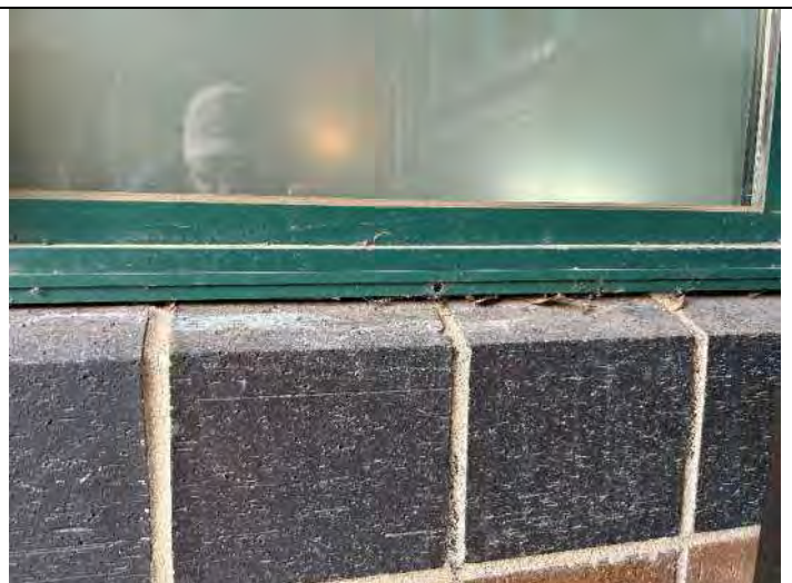
Elevation 9: No sealant below storefront window.
