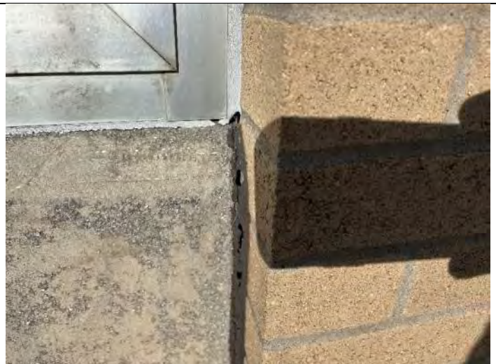
Elevation 9: Sealant at EIFS and window are failed.
