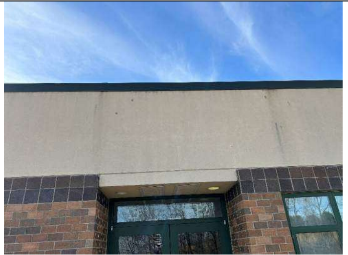
Elevation 2: Algae and woodpecker damage.
