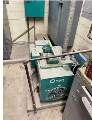
Figure 5- Existing Onan Emergency Generator
