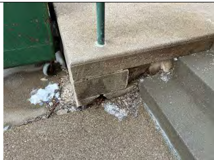
Elevation 6: Repair CMU loading dock.
