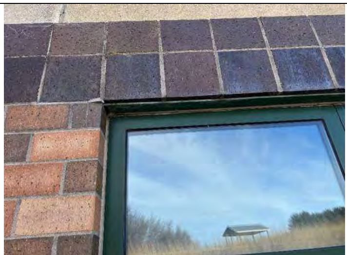
Elevation 3: Repair mortar at window head.
