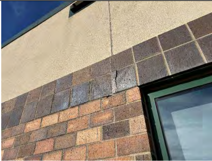
Elevation 1: Repair failed brick, seal control joint.
