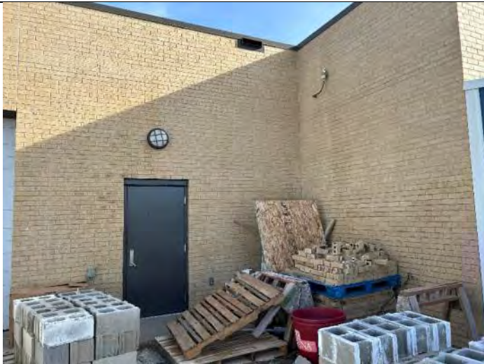
Elevation 4: HM door needs replaced and resealed.
