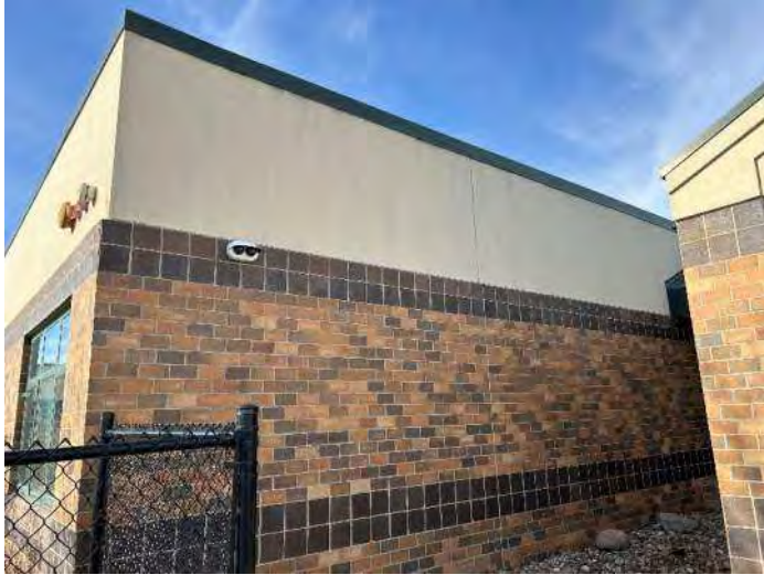
Elevation 11: EIFS is thin and needs cleaning.
