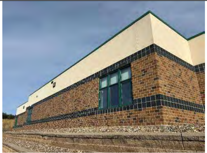
Elevation 7: Reseal control joints.
