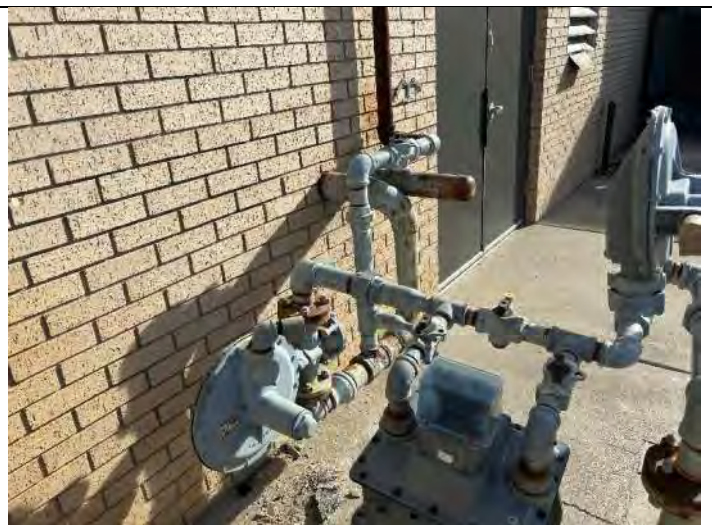
Elevation 6: Seal pipe penetrations.
