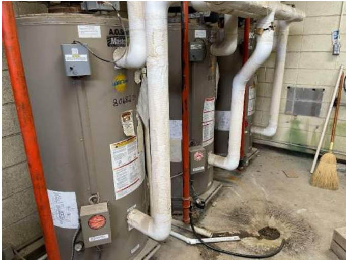
Figure 4- Domestic Water Heaters
