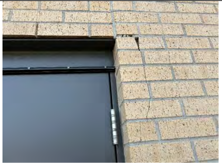
Elevation 11: Cracked brick at door head/jamb.
