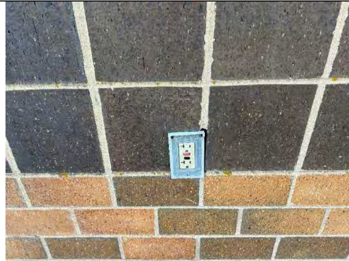
Elevation 2: Outlet needs cover and grout repair.
