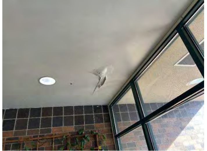
Elevation 11: Leak below roof transition above.
