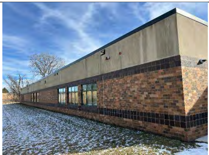
Elevation 3: Repair thin EIFS, reseal control joints.
