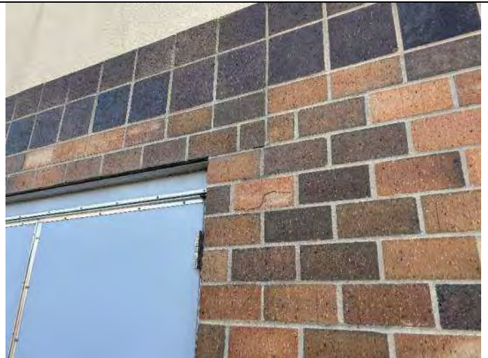
Elevation 5: Repair brick with broken face.
