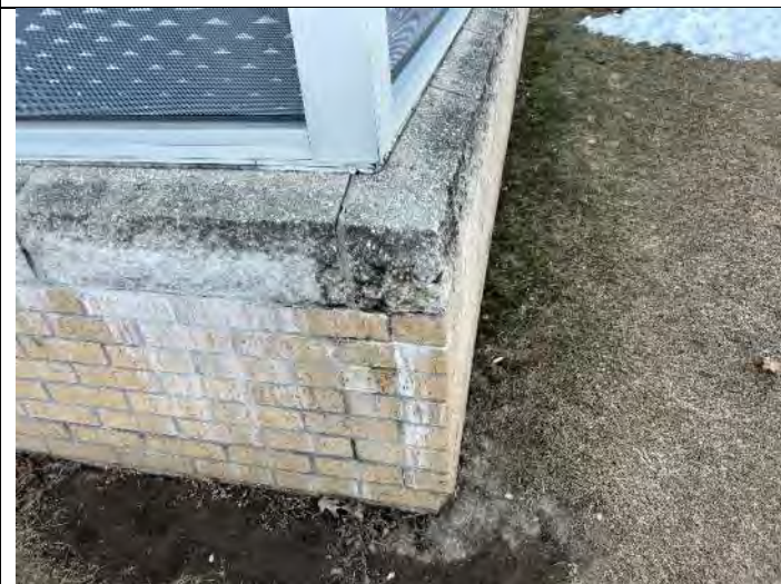
Elevation 12: Clean and seal brick and sill.
