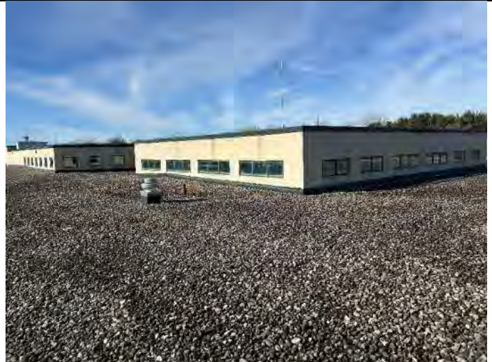
Elevation 12: EIFS is thin and needs cleaning.
