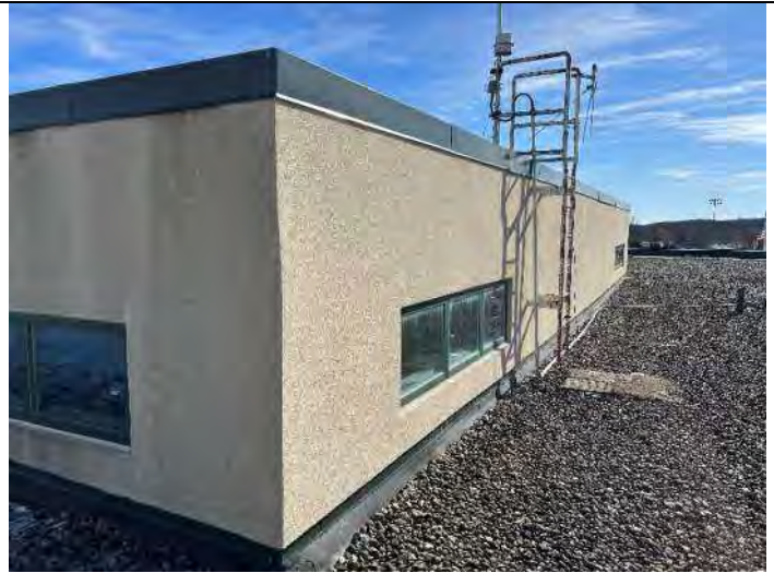
Elevation 13: EIFS is thin and needs cleaning.
