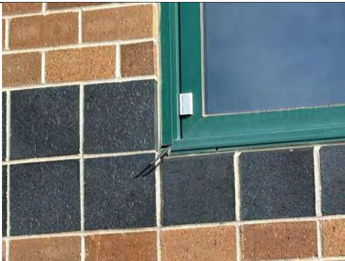
Elevation 7: Vinyl seals coming out of window.
