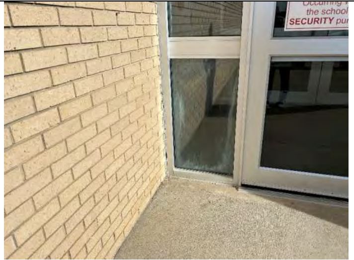
Elevation 6: Replace sealant at door frame.
