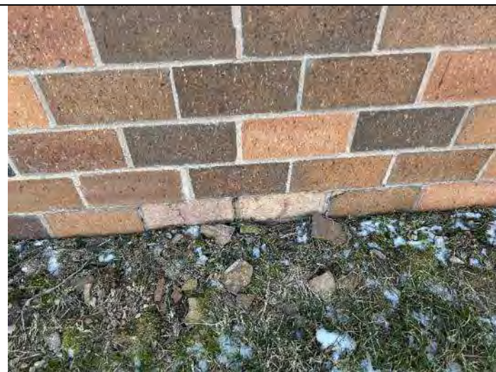
Elevation 3: Repair brick with spalling faces.
