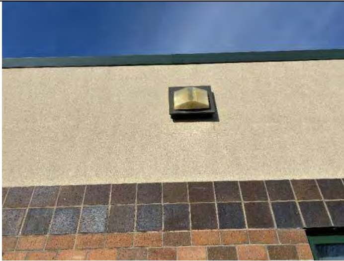
Elevation 10: EIFS repair needed below light.
