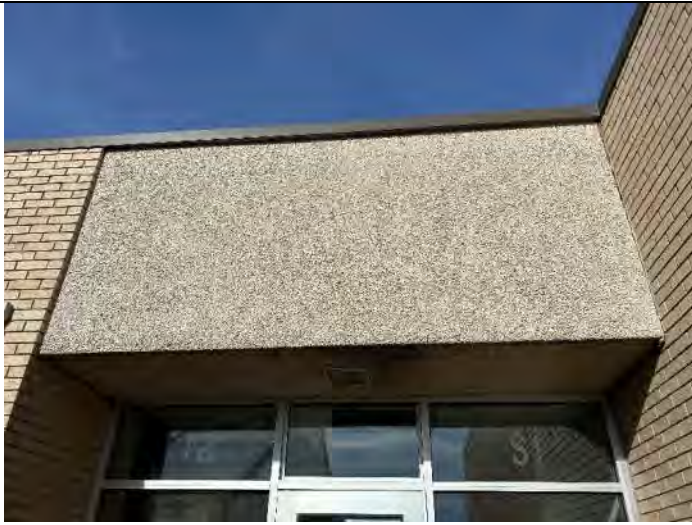
Elevation 7: Reseal stone panel and door frame. Resupport sagging framing of stone panel.
