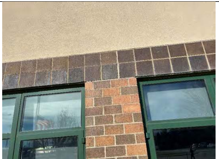
Elevation 1: Mortar failed between windows.
