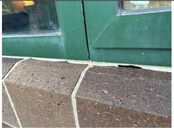
Elevation 10: Windows need resealed.
