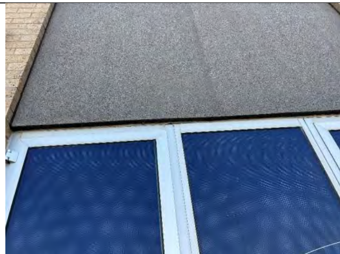
Elevation 3: New sealant required around windows and EIFS
