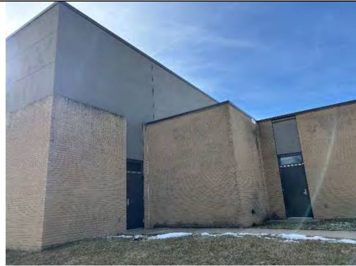
Elevation 2/3: EIFS failed, brick is algae stained.
