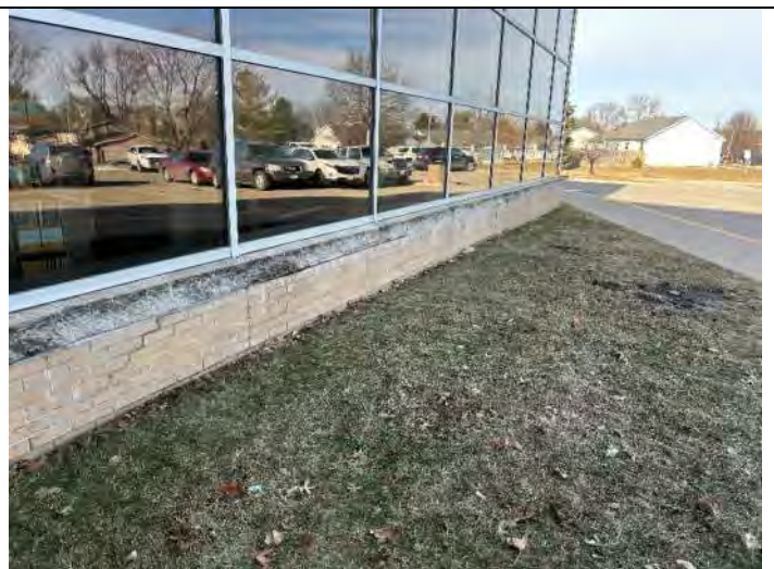
Elevation 12: Clean and seal brick and sill.
