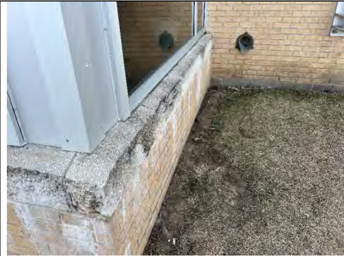
Elevation 12: Clean and seal brick and sill.
