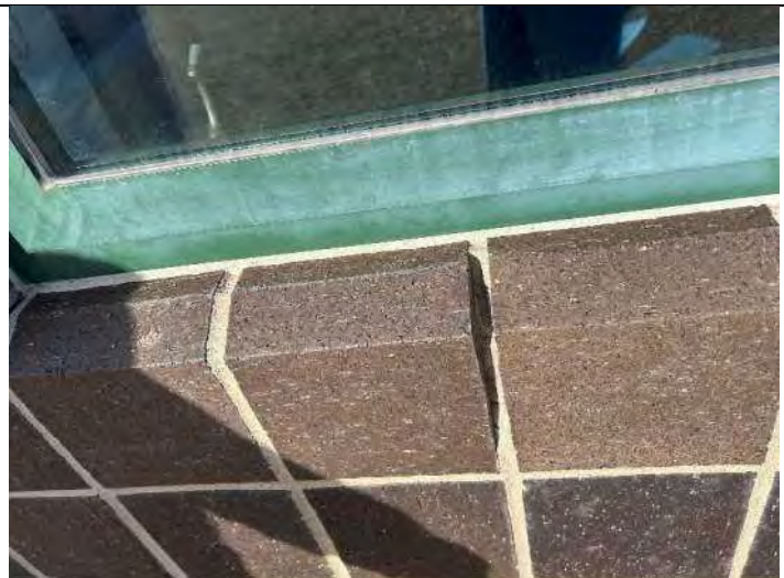
Elevation 3: Repair mortar, reseal windows.
