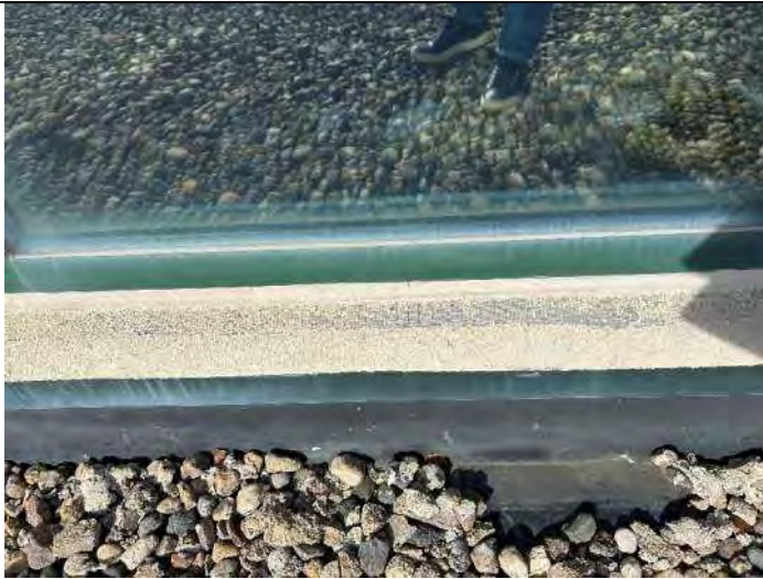
Elevation 12: EIFS sills are very thin.
