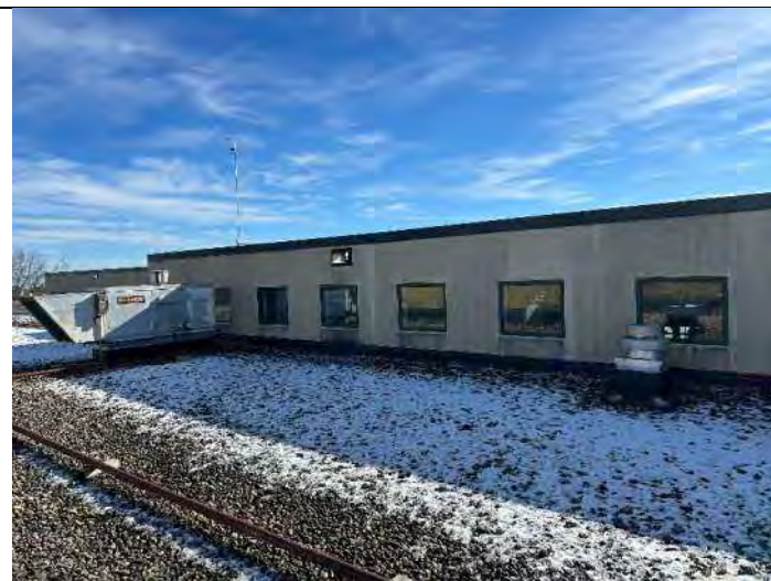
Elevation 12: EIFS is thin and needs cleaning.
