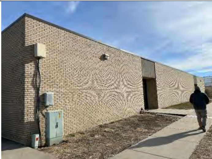
Elevation 7: No weeps in brick wall.
