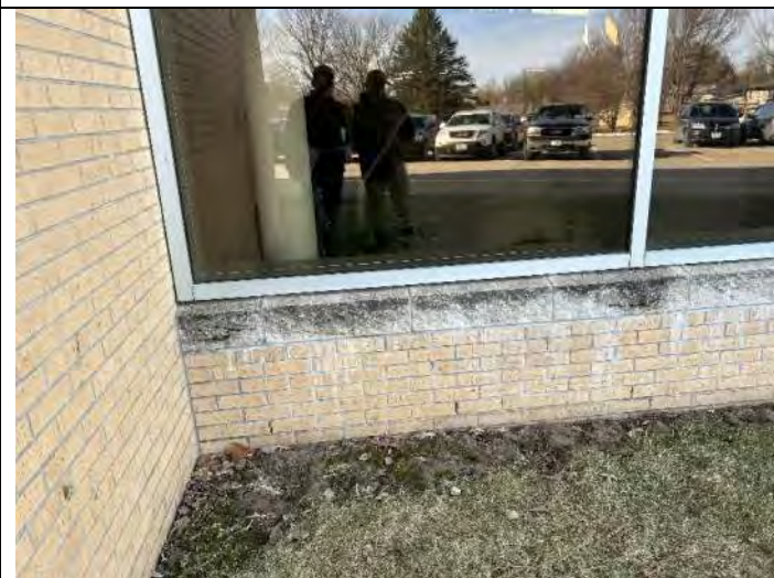
Elevation 12: Clean and seal brick and sill.
