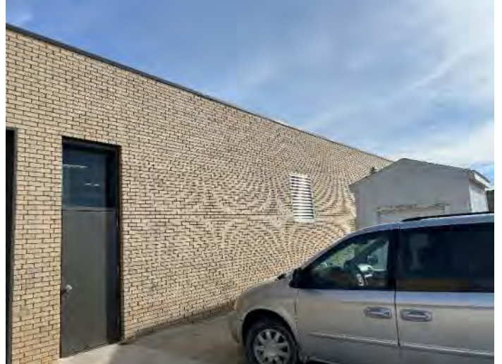
Elevation 5: Replace HM door.
