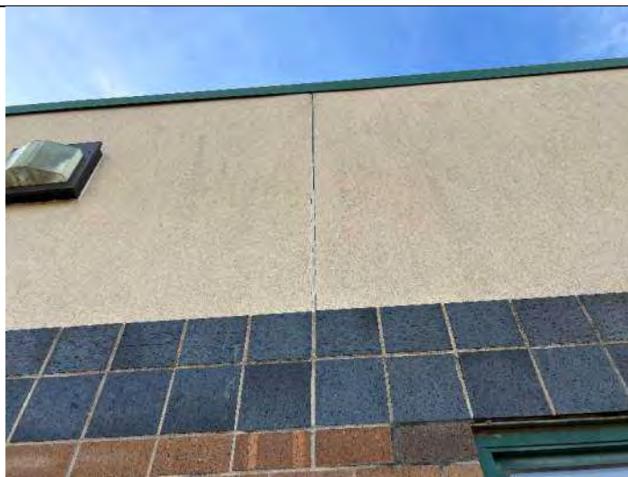
Elevation 9: Reseal control joints.
