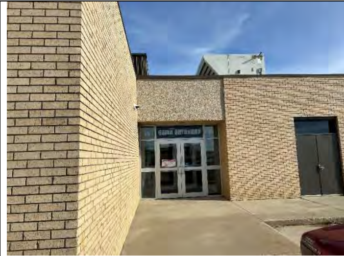
Elevation 5: Replace sealant at stone panel and door.
