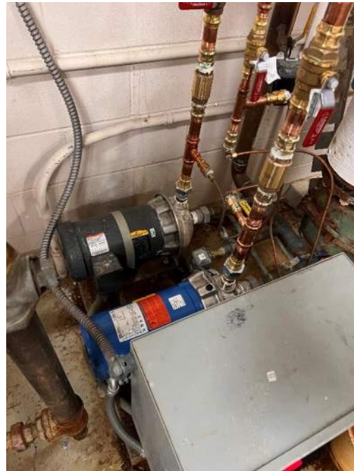
Figure 5- Domestic Water Booster Pumps
