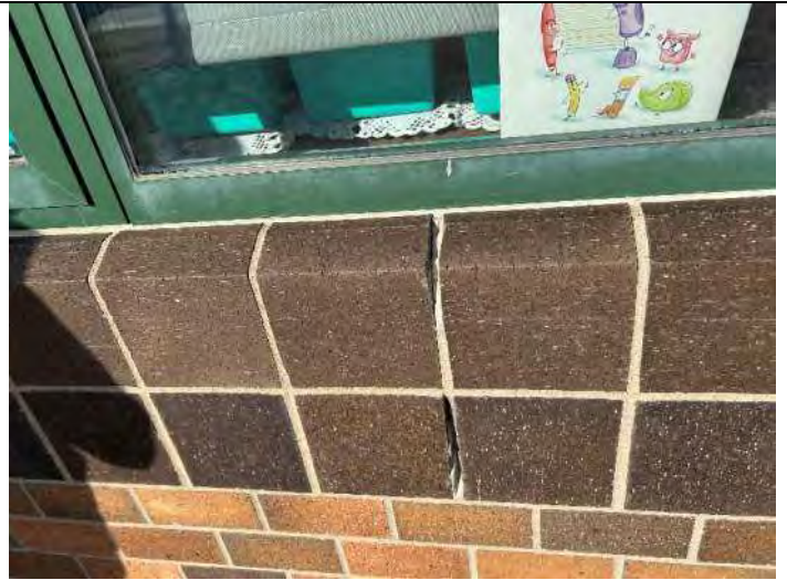
Elevation 1: Repair mortar, reseal windows.
