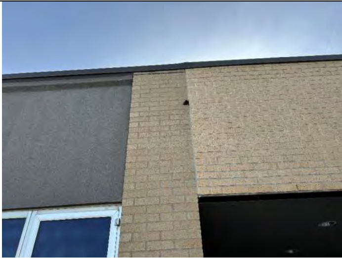
Elevation 3: Broken brick needs replaced.
