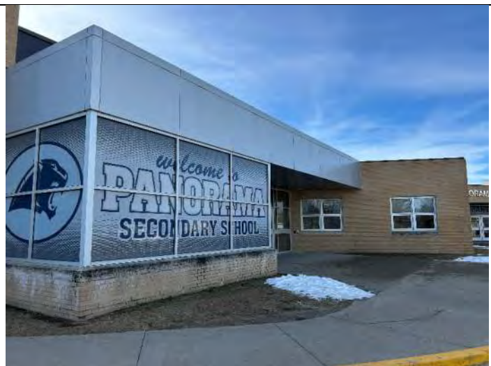
Elevation 12: Clean and seal brick and sill.
