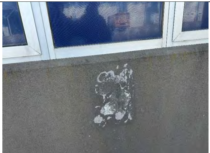
Elevation 3: EIFS needs repaired.
