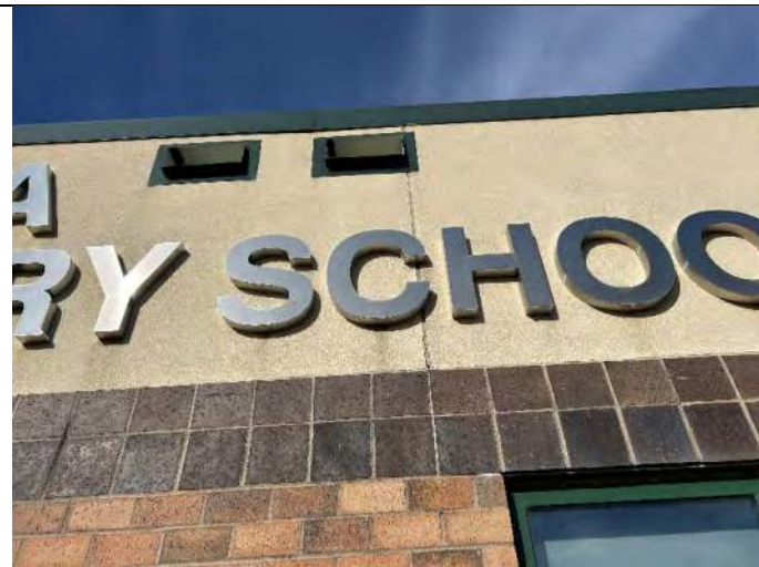
Elevation 1: Reseal control joints.
