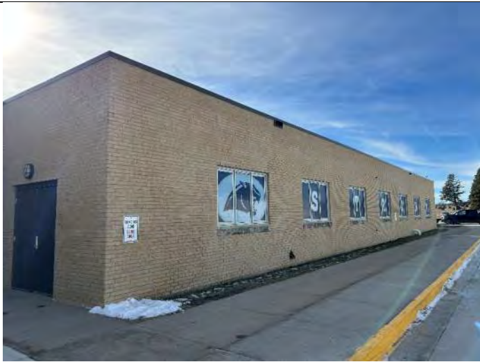
Elevation 4: Sill block is algae stained.
