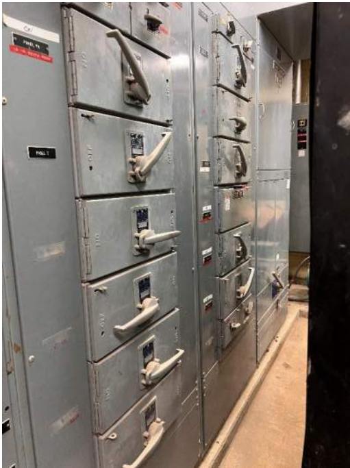
Figure 1 – Main Electrical Switchboard showing Boiler Encroachment at right
