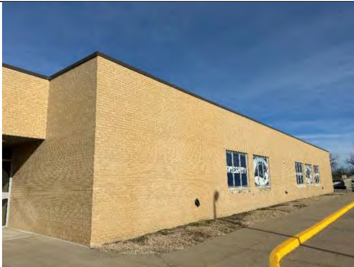
Elevation 10: Windows needs new sealant and sills cleaned .
