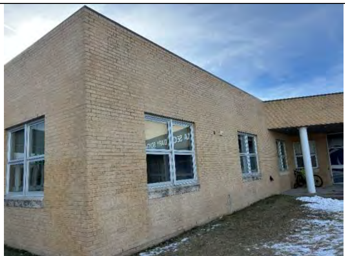
Elevation 12: Brick wall has moisture in it.
