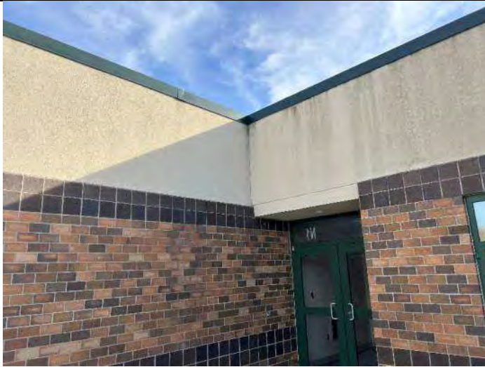
Elevation 4: Repair thin EIFS, reseal control joints.
