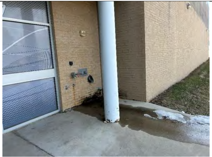
Elevation 1: Water/algae damage at FDC.
