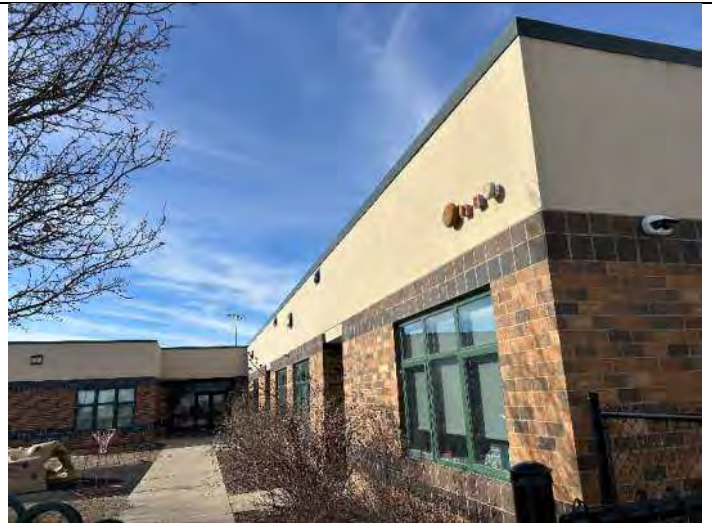
Elevation 10: EIFS is thin and needs cleaning.
