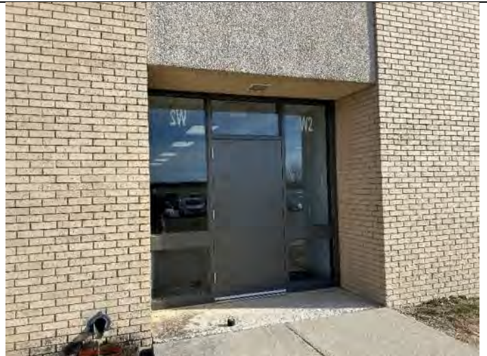
Elevation 7: Reseal stone panel and door frame.
