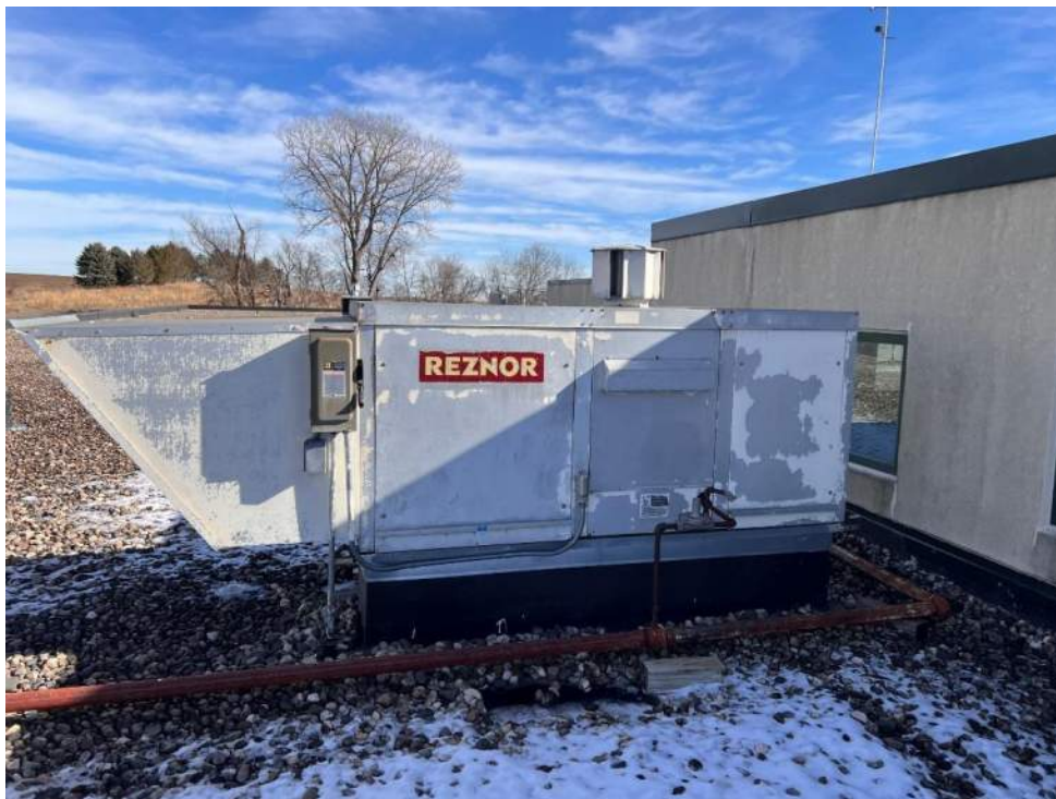
Figure 3 – Reznor Ventilation Make-Up Air Unit on Roof
