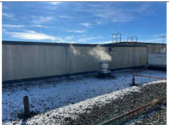
Elevation 12: EIFS is thin and needs cleaning.
