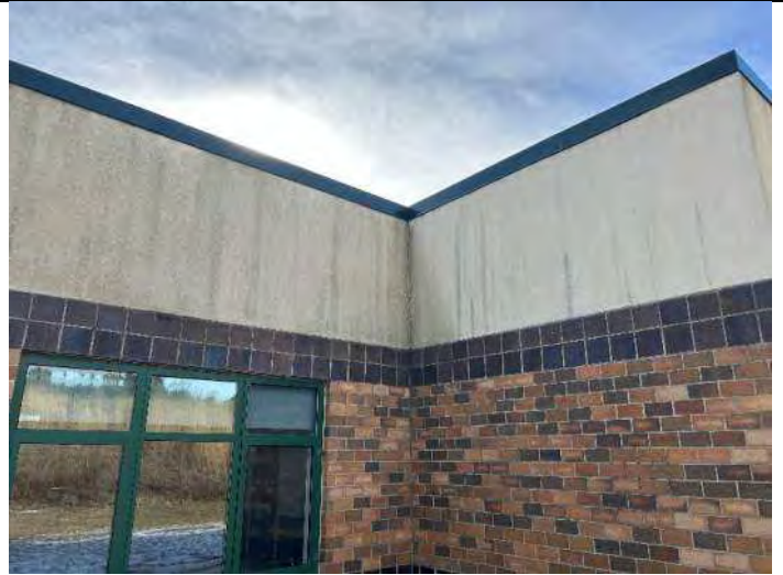
Elevation 4: Repair thin EIFS, reseal control joints.
