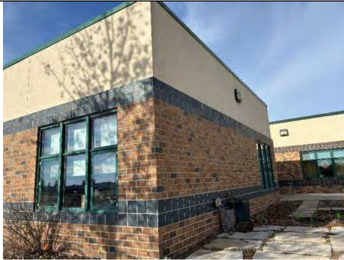
Elevation 7: EIFS is thin and needs cleaning.
