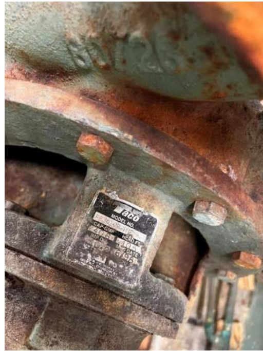
Figure 2- Close-up of Corrosion on Geo Pump
