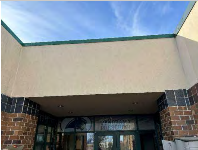
Elevation 10: Corner control joints need resealed.
